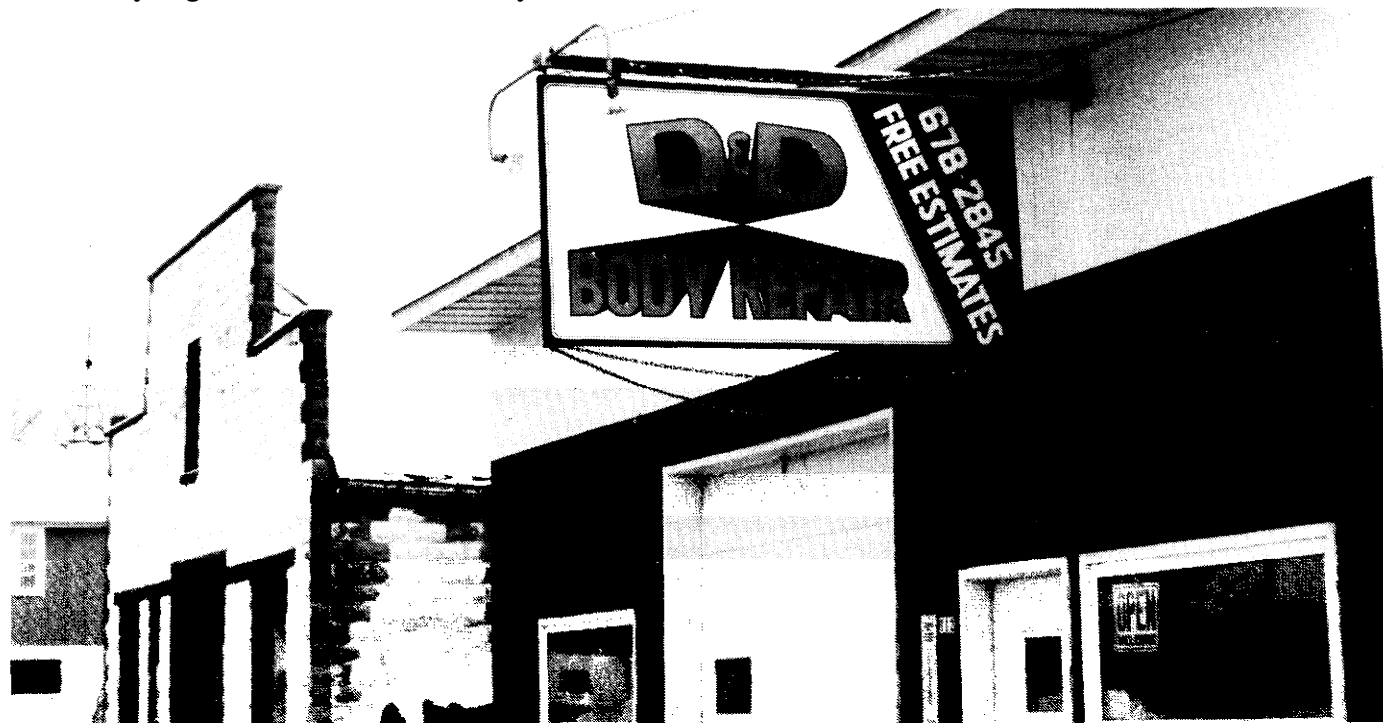
D&D Body Repair Shop Stetsonville, WI
